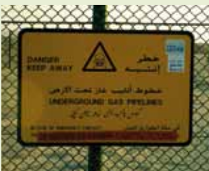
▼ Pipeline protection fence in the Middle East after 12 years.
