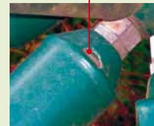
▼ No under-film corrosion after 12 years
