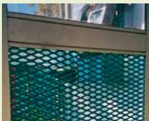
▼ PPA 571 coating still as new after 6 years.
