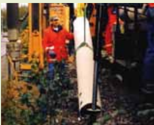
▼ Concrete reinforced piles in Scandinavia.
